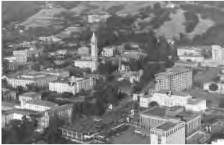
FIGURE 3.1. An aerial view of the UC Berkeley, 1965. The campus expanded rapidly southward (to the right in this picture) in the postwar period, stretching beyond Sather Gate (# 4). The complex of buildings labeled #1 are the student union buildings built in the early 1960s. #2 is Sproul Hall, now part of the Berkeley campus; Sproul Plaza is #5. The plaza the Berkeley administration wanted to designate as the “Hyde Park area” is below #1 in this picture. Photograph originally published in Heirich (1971).
