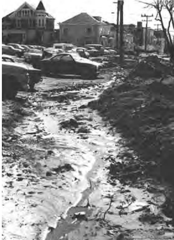
FIGURE 3.8. The muddy parking lot (lot 1875-2) that eventually became People's Park. Photograph by Mark Harris.
